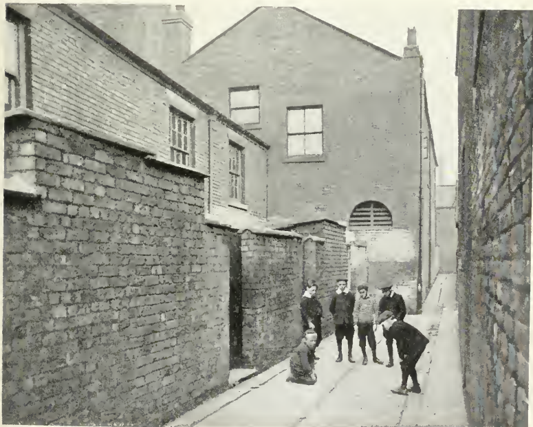
WORKSHOP (GABLE END ON) OFF KIRBY STREET, ANCOATS, MANCHESTER, WHICH WAS THE PUBLIC HALL AND PLACE OF GOOD FRIDAY CONFERENCE, APRIL 3RD, 1863 (see page 29).
